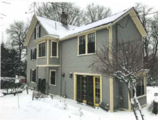
1.3 rear / partial north elevation
