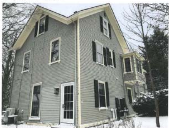
1.2 rear / partial south elevation
