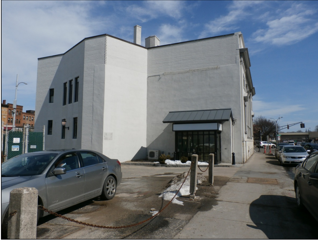
Above: West elevation of 160 Washington Street
