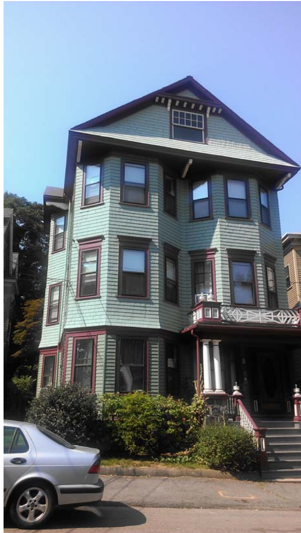
5 Irving Street Front Façade
