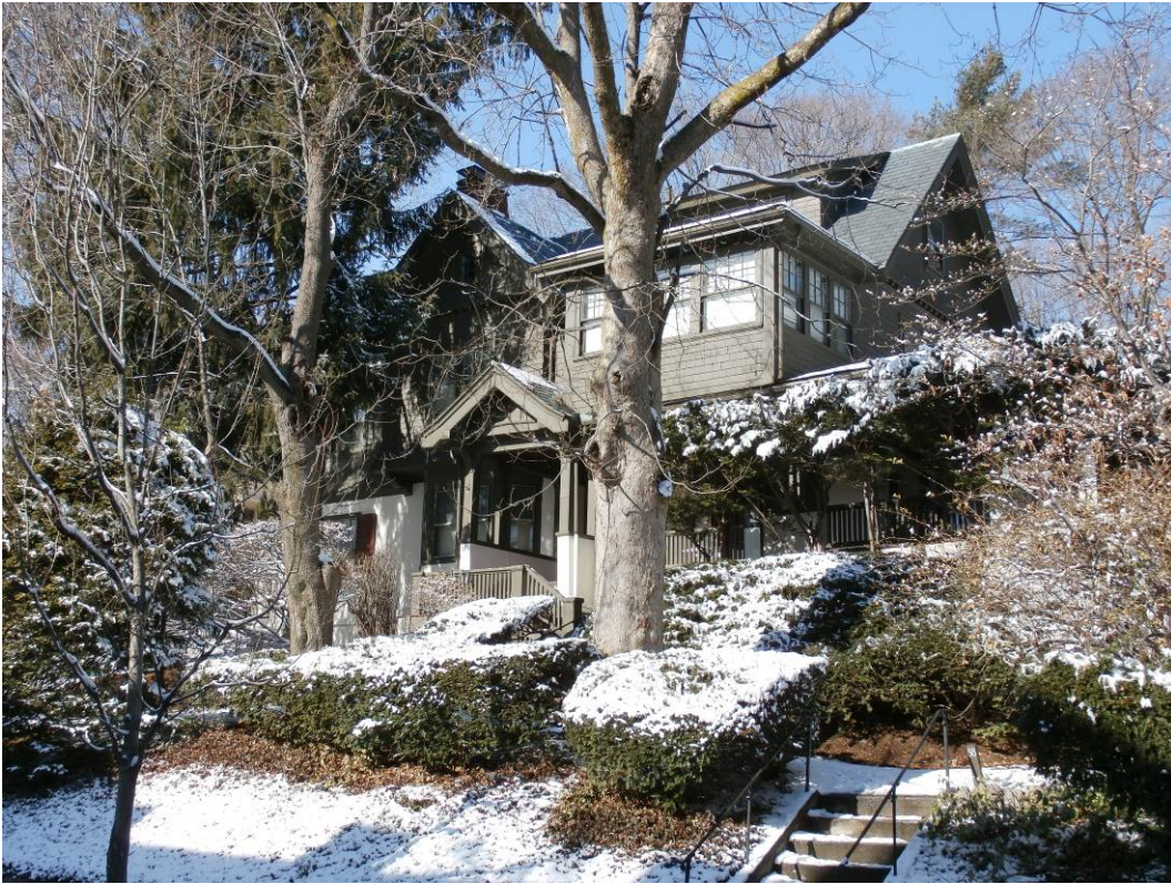
88 Mason Terrace Front Façade
