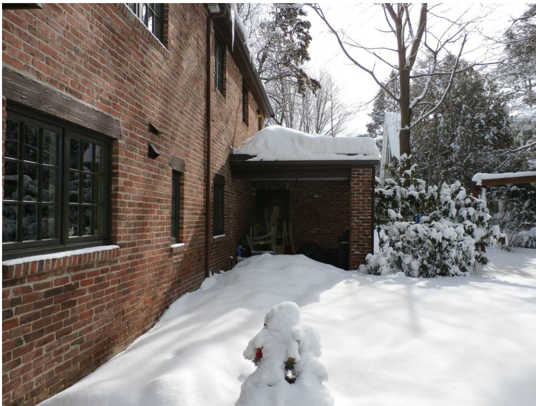
Unenclosed porch and area for second story addition
