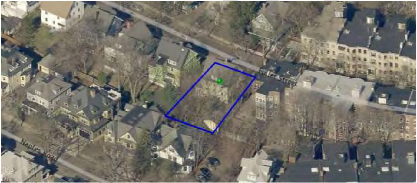
Aerial view of 123 Fuller Street, looking west.
