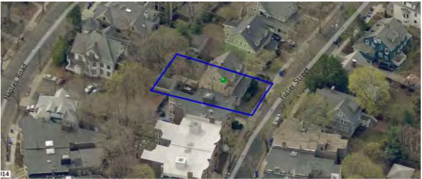
Aerial view of 123 Fuller Street, looking south.
