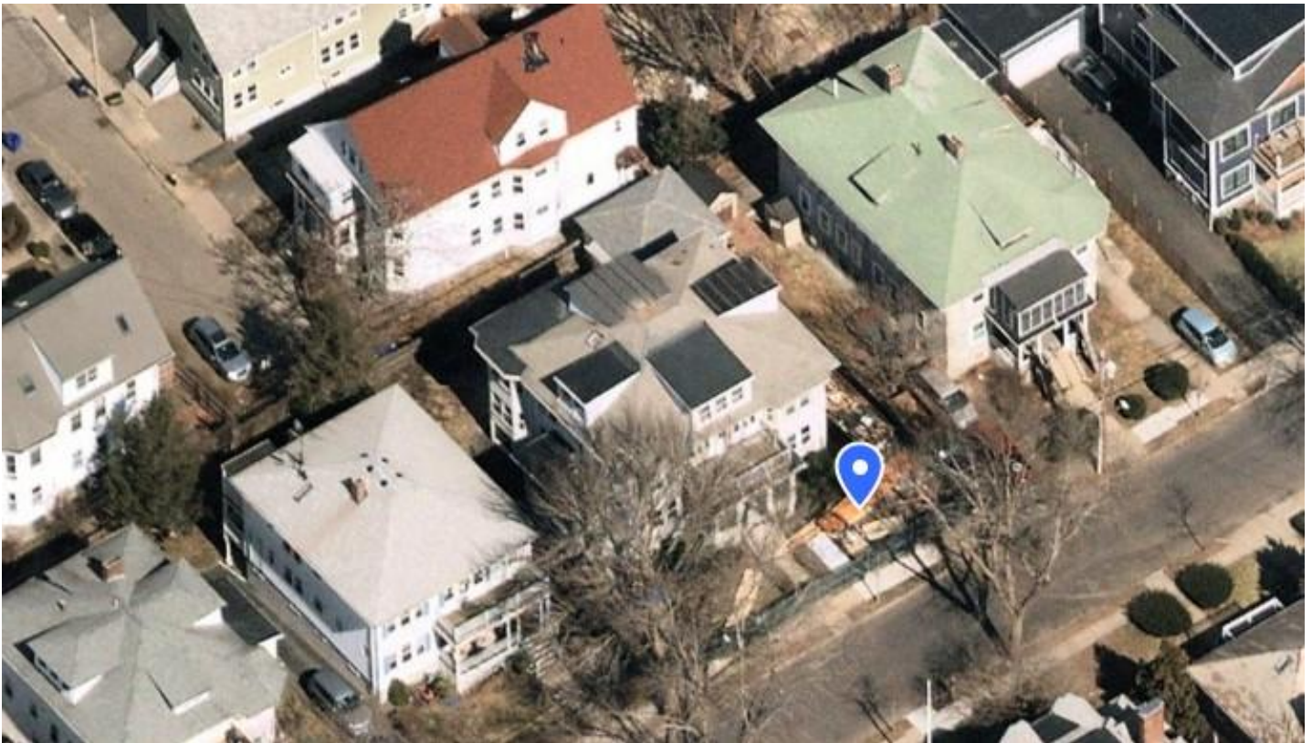
Aerial view of 49 Verndale Street, looking north.
