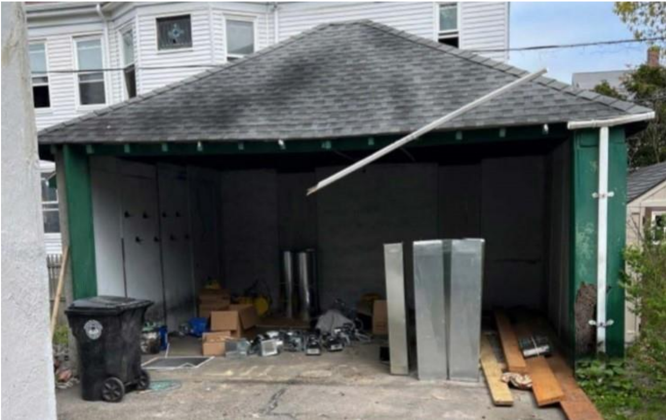
Photograph of the front of the garage at 49 Verndale Street
