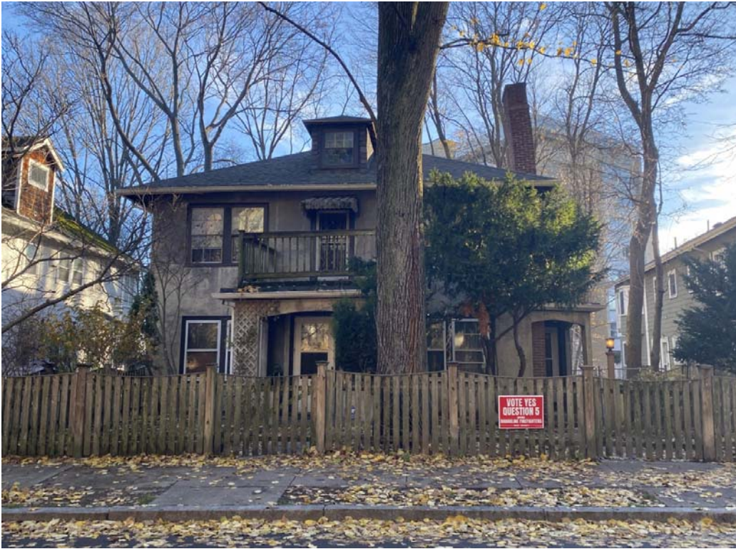
View of front façade; 59-61 Mason Terrace; taken by staff December 2022
