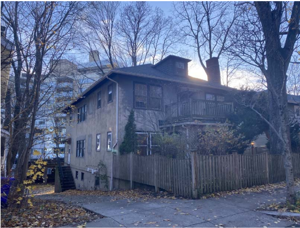
View of left façade; 59-61 Mason Terrace; taken by staff December 2022
