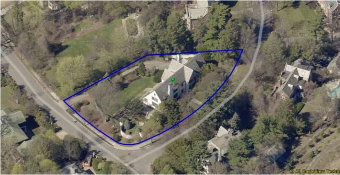
Aerial view of 161 Hyslop Road, looking north.
