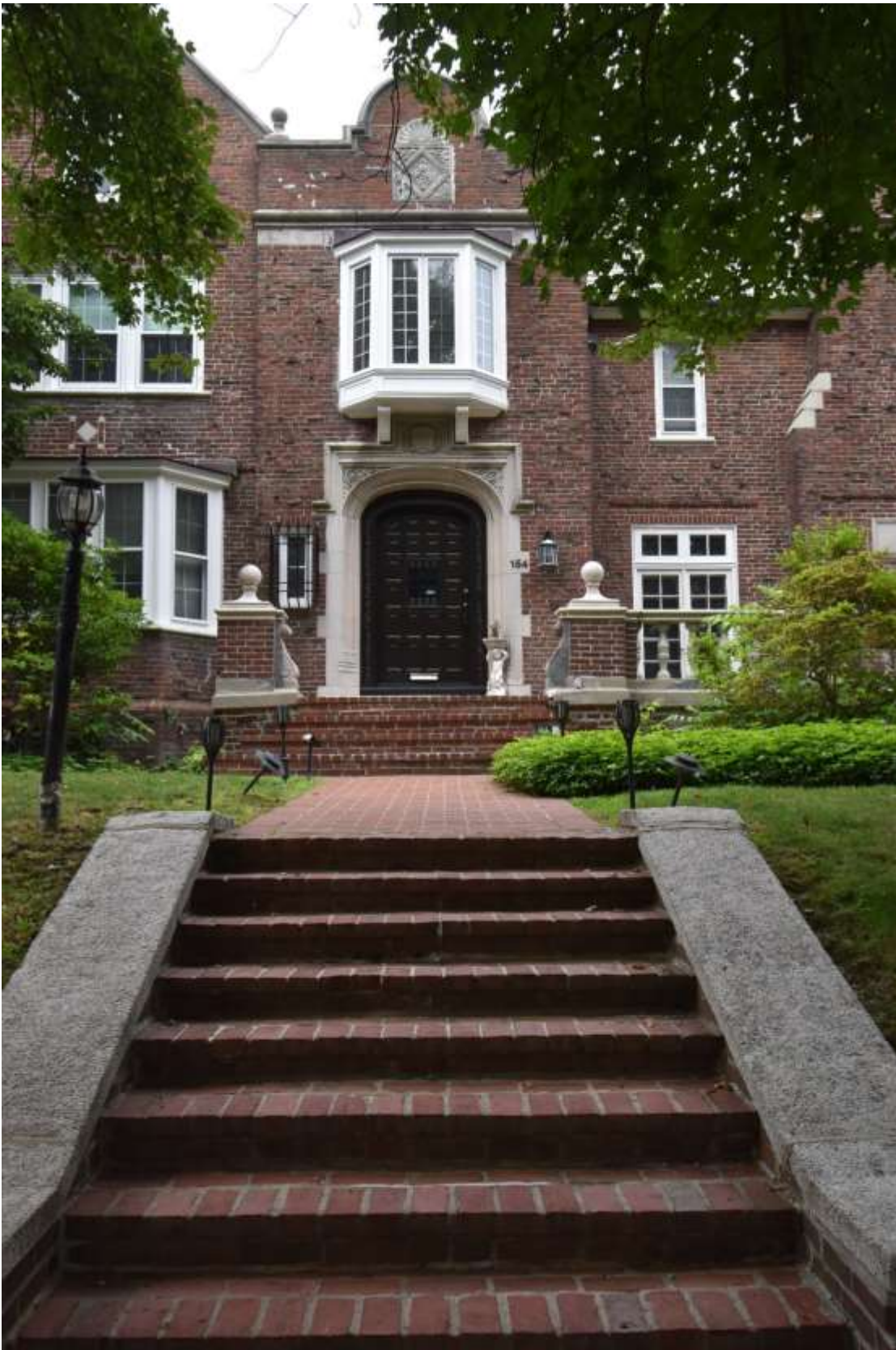
154 Hyslop Road, similar crest above the front entrance
