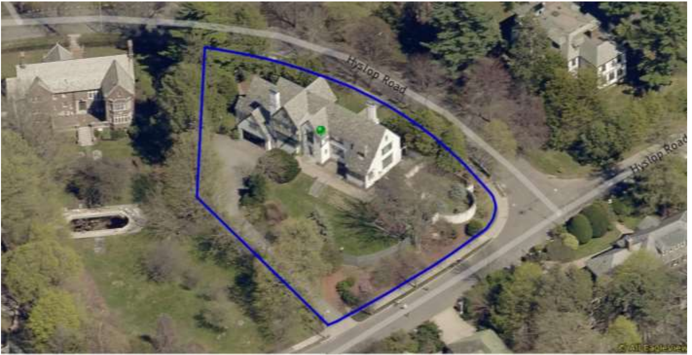
Aerial view of 161 Hyslop Road, looking east.
