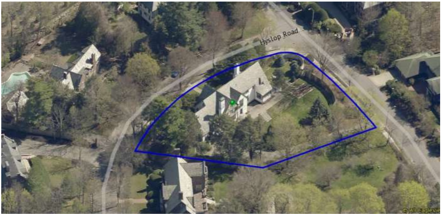
Aerial view of 161 Hyslop Road, looking south.
