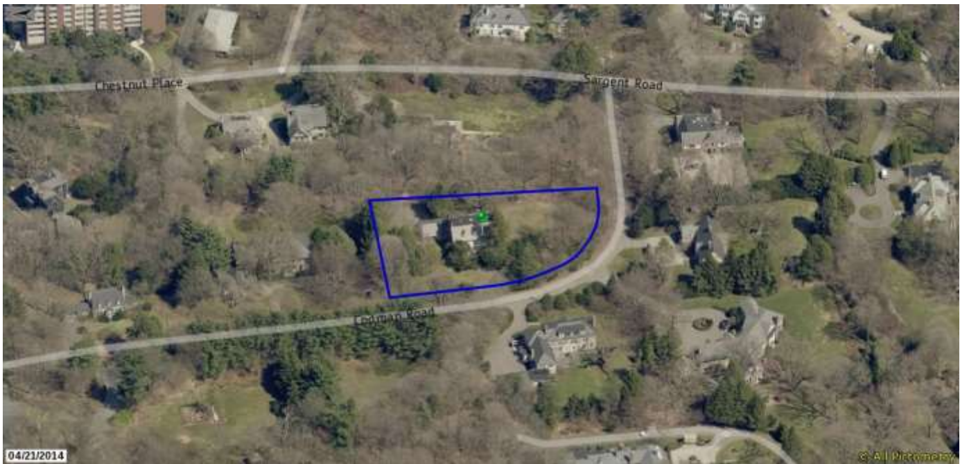
Aerial view of 41 Codman Road, looking east.
