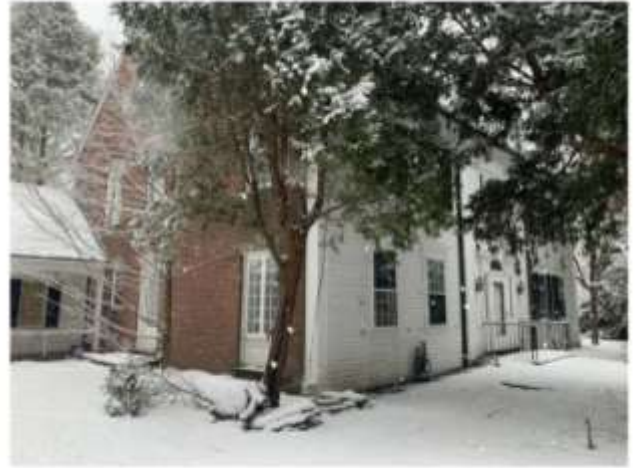
GARAGE & MAIN HOUSE - NORTHWEST CORNER
