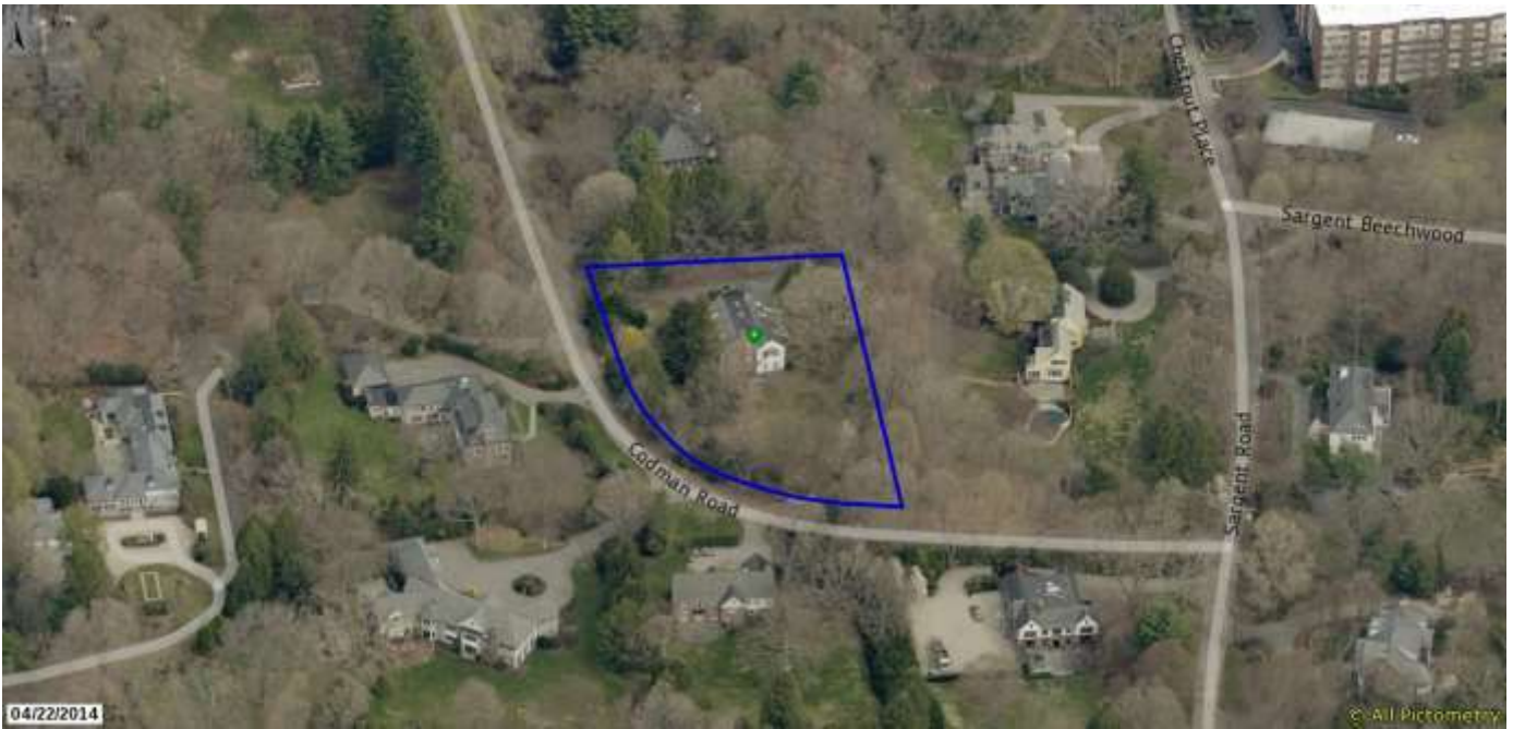
Aerial view of 41 Codman Road, looking north.
