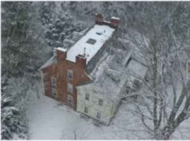
AERIAL - SOUTHEAST VIEW
