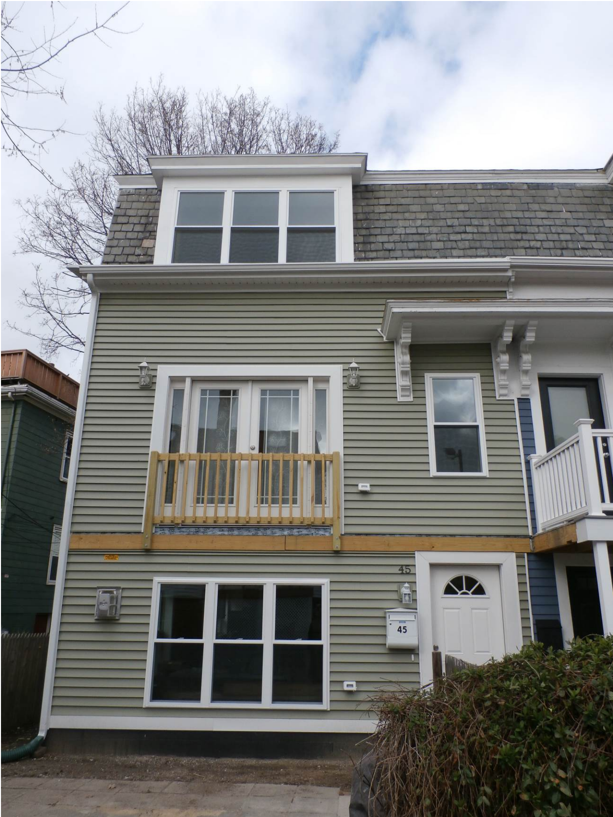
Existing area on second floor for porch
