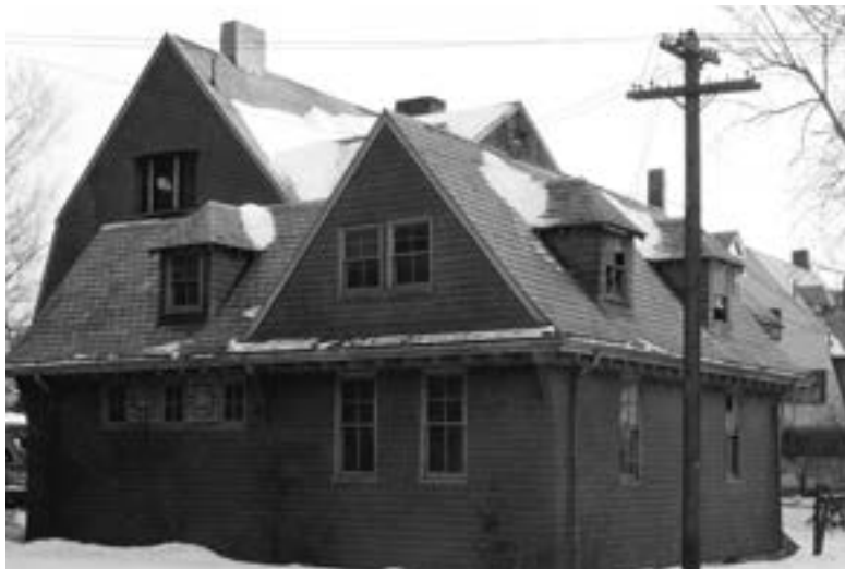
1936 Photo of carriage house north elevation
