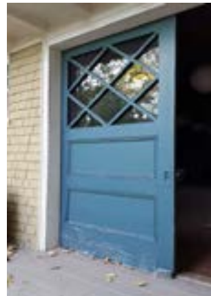
Existing south elevation rolling barn door that will be recreated for east elevation
