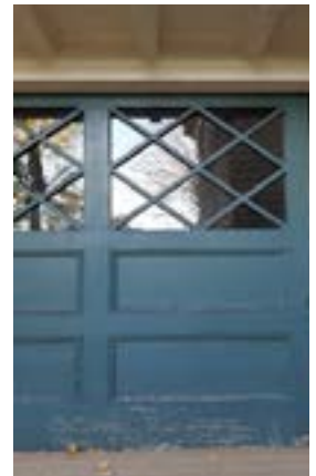
Existing south elevation rolling barn door that will be recreated for east elevation
